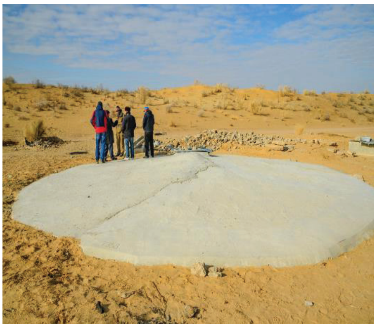
D) Restored sardobs (after project implementation)
