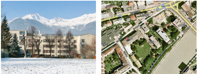
Fig. 5.1: Hötting Secondary School, Innsbruck
