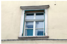
Fig. 1.18: The latest prototype installed in the Waaghaus
