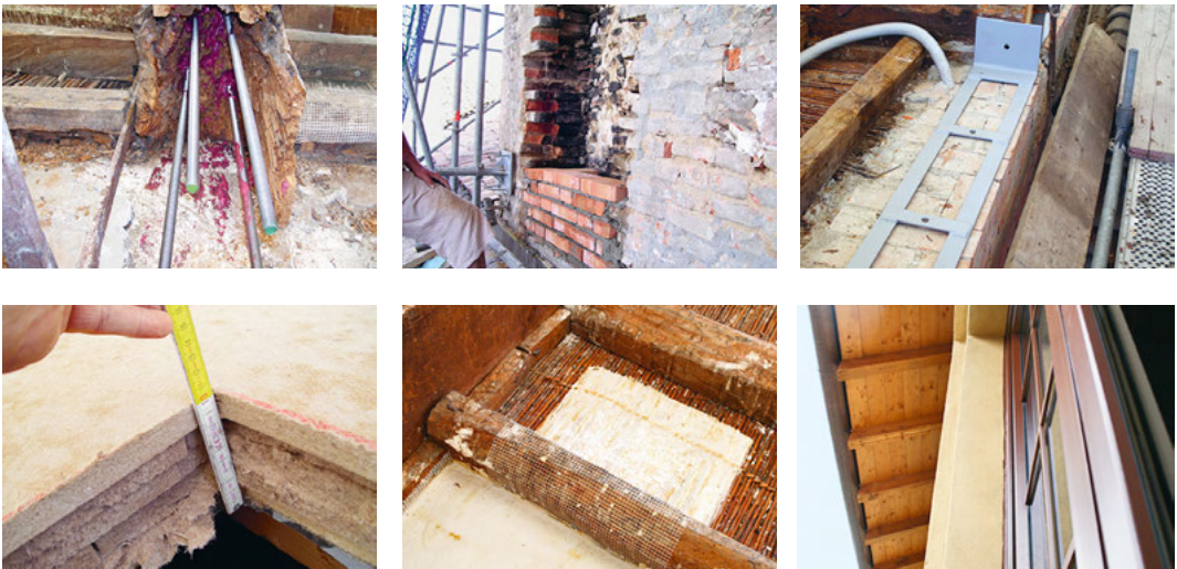
Fig. 2.11: Images of the roof refurbishment, structural consolidation, and ceiling renovation
