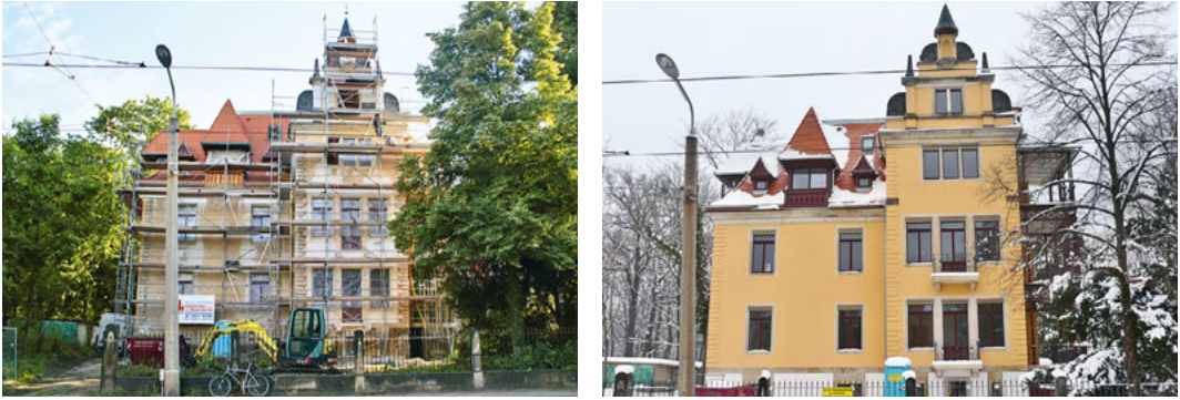
Fig. 6.6: Wilhelminian style building in Dresden, before and after renovation
