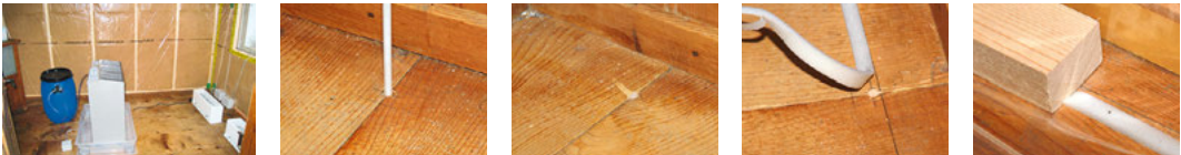
Fig. 8.6: Installation of the internal insulation
