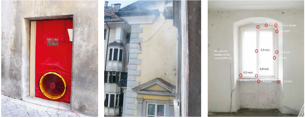
Fig. 1.9: Fan installed in the entrance door; gas overflow through window; measurement of air velocity at a pressure difference of 50 Pa at several points of the existing window. The blower door test for the building resulted in nearly 10 1/h, value
