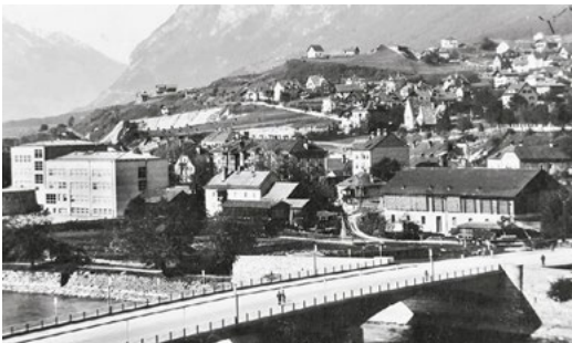
Fig. 5.5: Rural environment (school at left of photo), viewed from south-east and site plan
