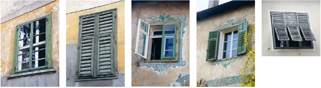
Fig. 3.14: Windows in Bolzano, Italy: Wooden shutters for shading in summer are exchangeable with winter windows. Their small frames allow optimal light access to the building. Shutters can be partly open for ventilation and light, but ensure also minimum ventilation and light through wood slats.
