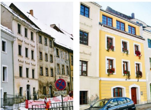
Fig. 6.13: Baroque building in Görlitz, before and after renovation
