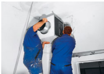
Fig. 5.16: Mounting of the fan box (left), the textile diffuser (middle) and the overflow silencer (right)
