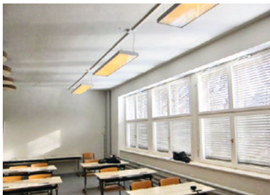
Fig. 5.11: Daylight redirection to the ceiling by the upper part of the blinds and sun-blocking by the lower part help to enhance daylight autonomy without glare problems
