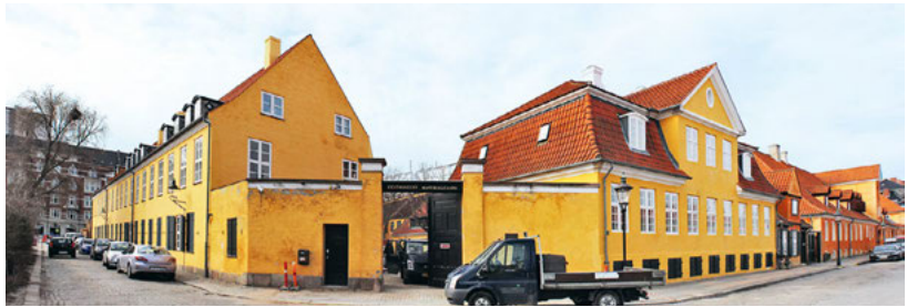
Fig. 4.1: Material Court of the Fortress
