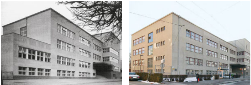
Fig. 5.3: View from Furstenweg (left: as built in 1931, right: status quo in Jan. 2011). In the years following WW2, the school was enlarged on the eastern side.
