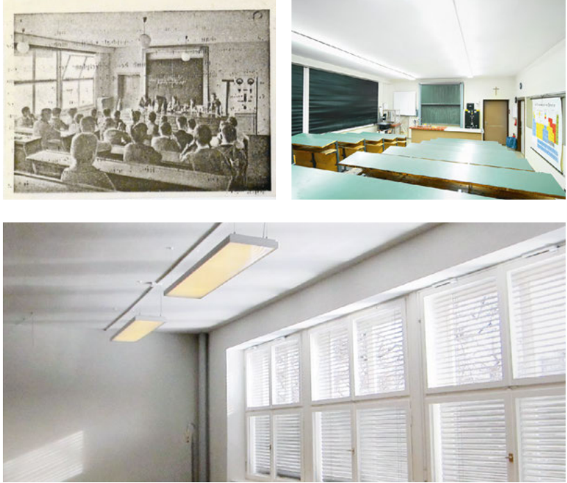
Fig. 9.5: Original incandescent light bulb (left); fluorescent tube - old technology (right) and LED technology (bottom)
