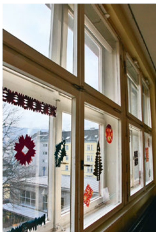
Fig. 9.3: CS5, Box-type window before intervention: l-r, both panes opening to the inside (view from inside); vertical cross section; original photograph from the outside, upper pane opening to the outside
