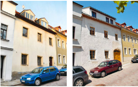
Fig. 6.16: Renaissance building in Freiberg, before and after renovation
