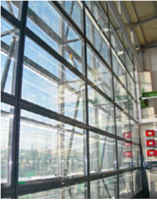
Fig. 5.68: Integration of PV in a glass facade
