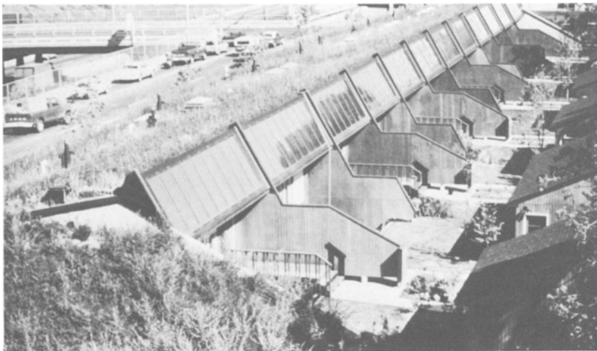
Fig. 6.3: Seward Town Houses—Minneapolis, Minnesota. Architect: Mike Dunn, Close Associates.
