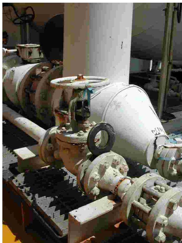
Figure 33: Spectacle blind in closed position
