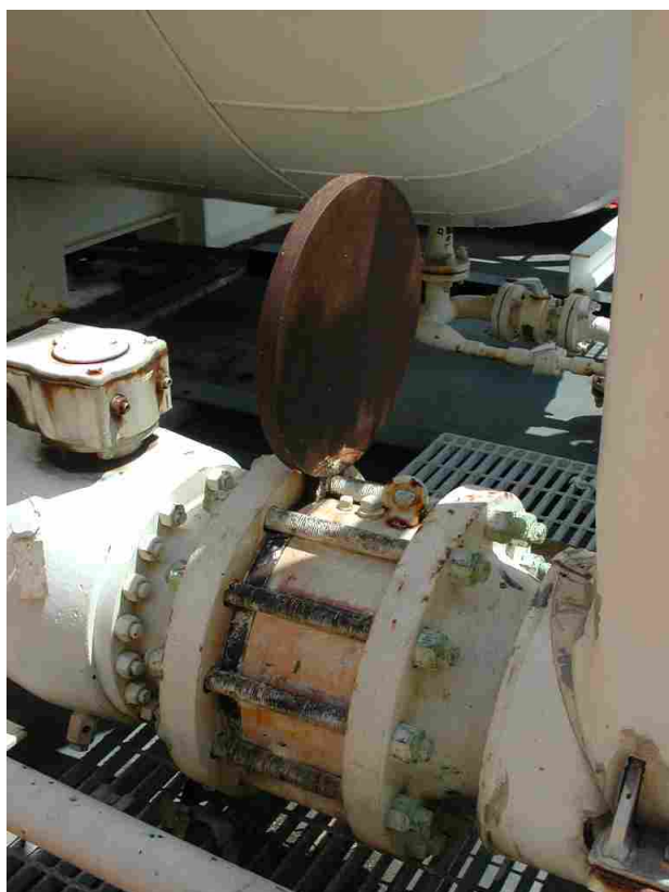
Figure 32: Spectacle blind in open position
