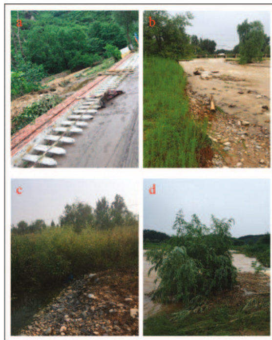
Figure 1. The protection measures damaged by the flood. (a) Destroyed retaining wall; (b) collapsed riverbank; (c) the living brush mattress measure before the flood; (d) the living brush mattress measure during the flood.
