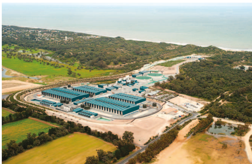
Figure 2. SSDP, general view. Source: Water Corporation.
