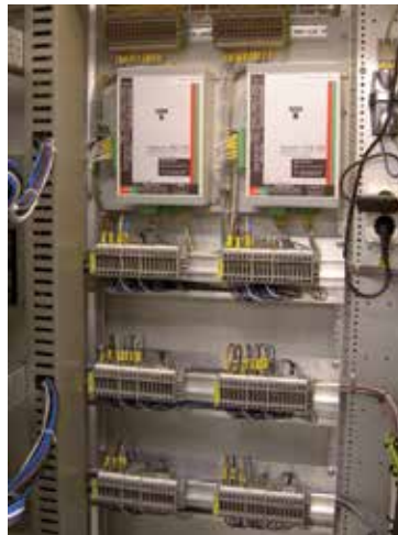
Fig. 8. PQ measurement devices installed in a substation (Source: Metrum)
