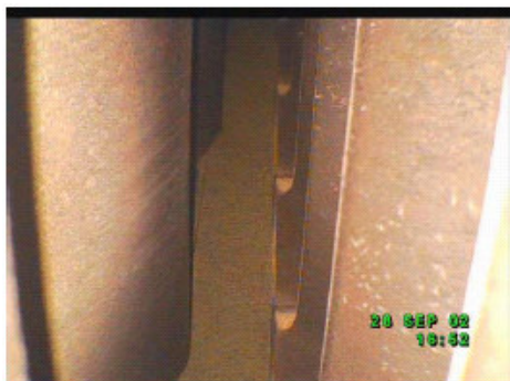
Corrosive deposits on Suction side of Rotor blade & Pressure side of Stator vanes.
