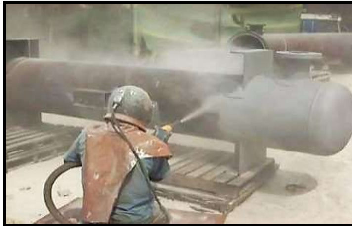
SSPC-SP5/NACE 1: White Metal Blast Cleaning
