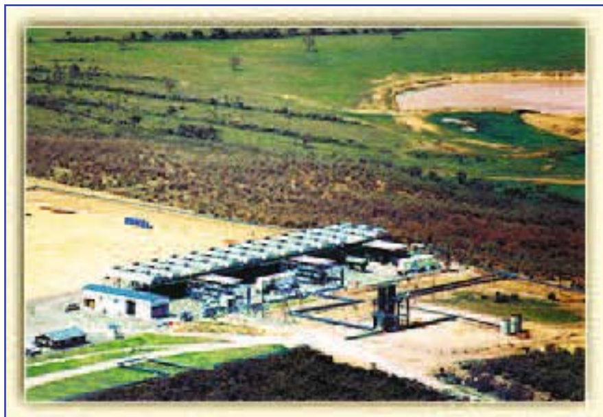
Fig. 2.2. Olkaria Geothermal Power Station in Kenya
