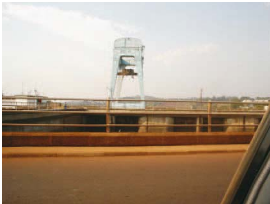
Fig. 3.2. Hydro power station at Owen Falls on river Nile in Uganda
