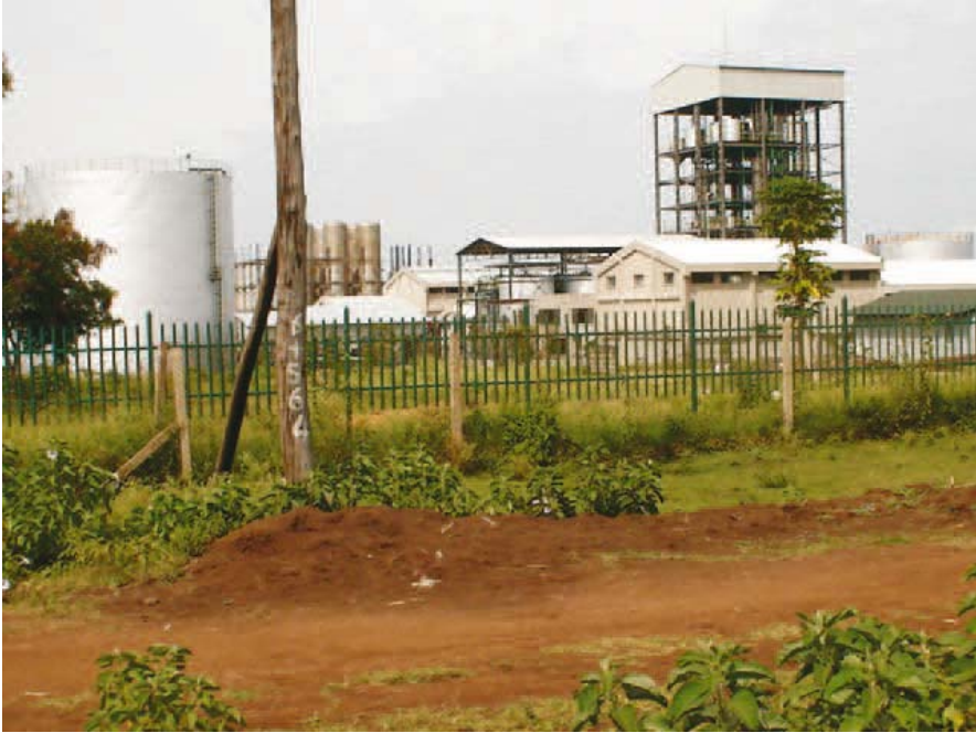
Fig. 3.4. Kisumu Molasses plant with un-tapped co-generation potential
