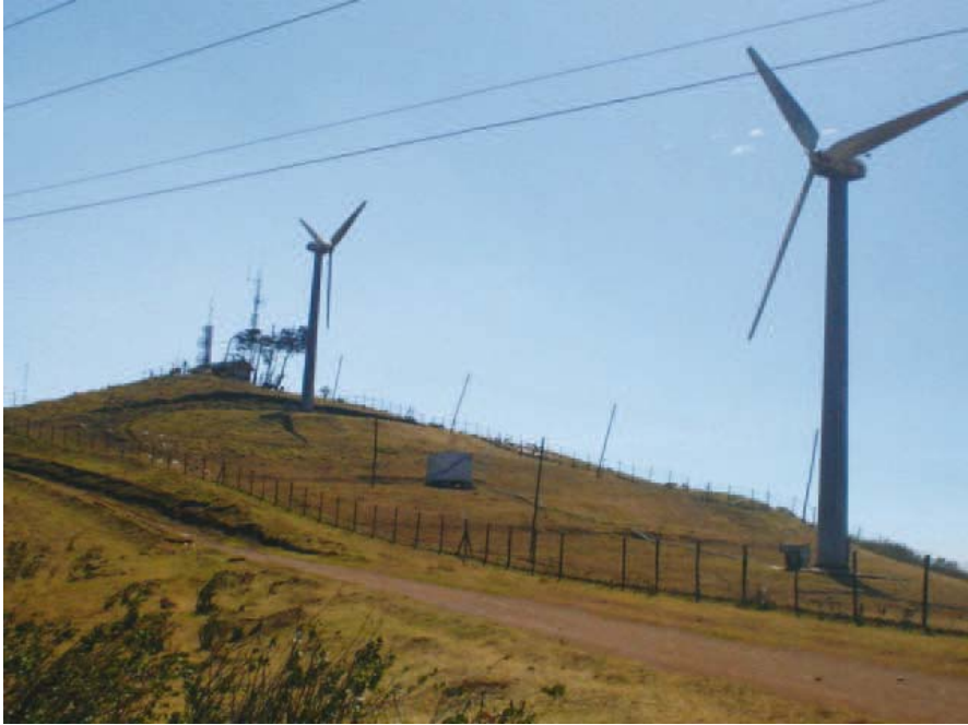
Fig. 3.6. Wind generator operating in Kenya (Ngong Hill)
