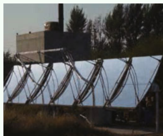
Fig. 3 Trough concentrator developed by the Institute of Electrical Engineering, Chinese Academy of Sciences
