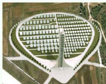
Fig. 5 Panorama of 1MW solar tower plant in Yanqing county, Beijing
