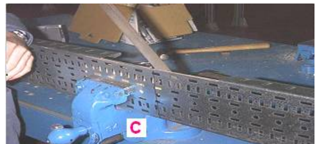
Figure 99: Construction of a flat 90° bend (C)
