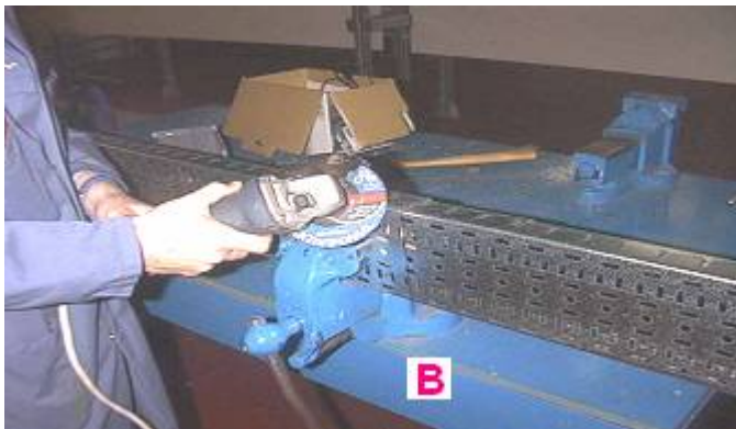
Figure 98: Construction of a flat 90° bend (B)
