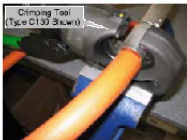
Figure 145: Place the connector in the crimping tool
