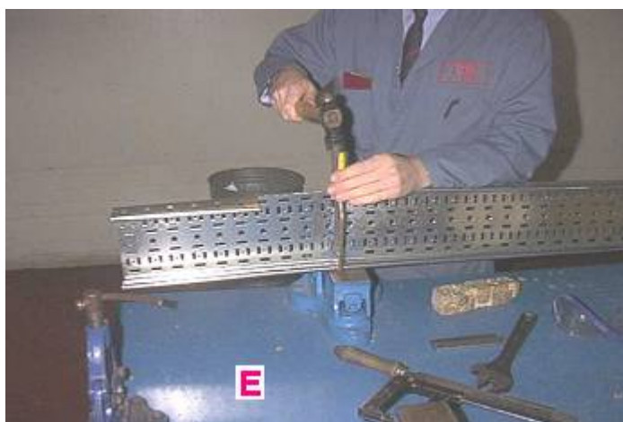
Figure 101: Construction of a flat 90° bend (E)
