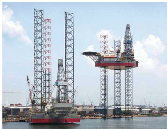
Jack-Up Drilling Rig
