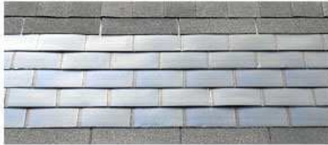
Figure 10-7 Building-integrated PV roofing.
