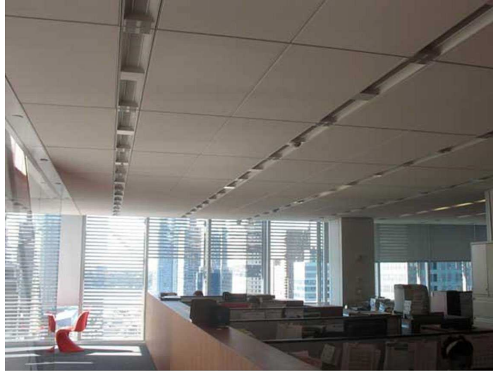
Figure 11-3 Interior view of the Times Building five years after occupancy. The overhead lighting is dimmed in response to available daylight, while the automated shades are adjusted to control for glare and direct sun.
