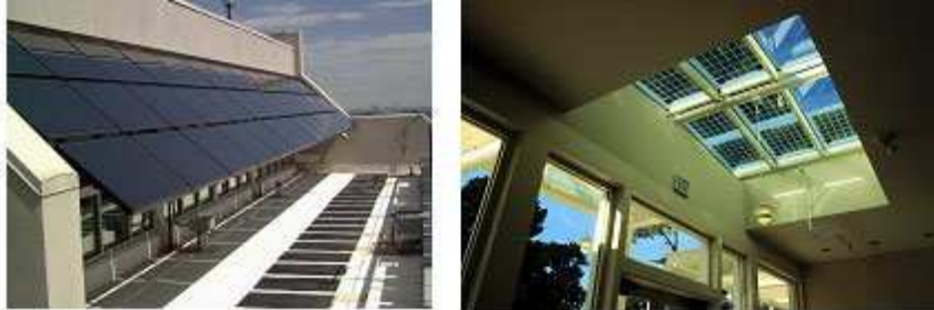
Figure 10-6 Building-integrated PVs.
