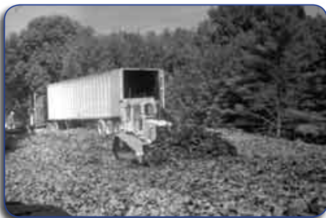
Exhibit E-2. Caterpillar D-4 spreading TDA for lightweight embankment fill at Portland Jetport Interchange
