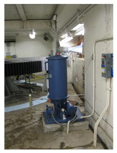
Figure 8-3. Automatic Grease-Dispensing System for Lock Machinery and Miter Gate Pintle
