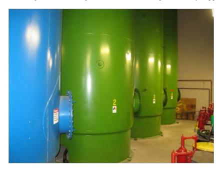
Figure 8-1. Hydroelectric Plant Turbine Oil Storage Tanks.
