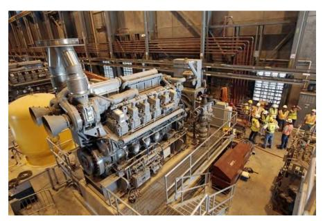
Figure 7-1. Diesel Engine for Pump Drive.
