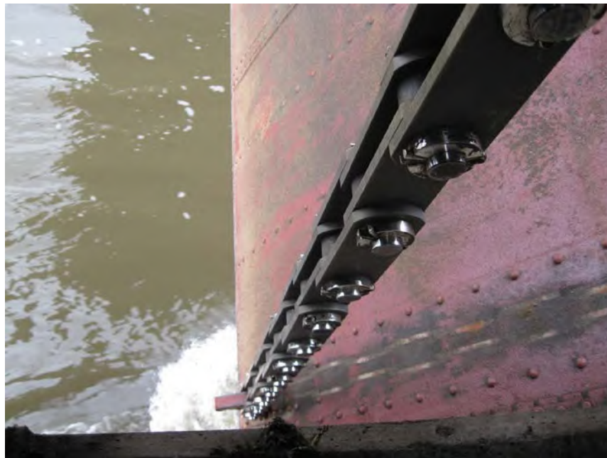
Figure 16-6. New Roller Chain Using Stainless Steel Pins and Aluminum Bronze Sidebars.
