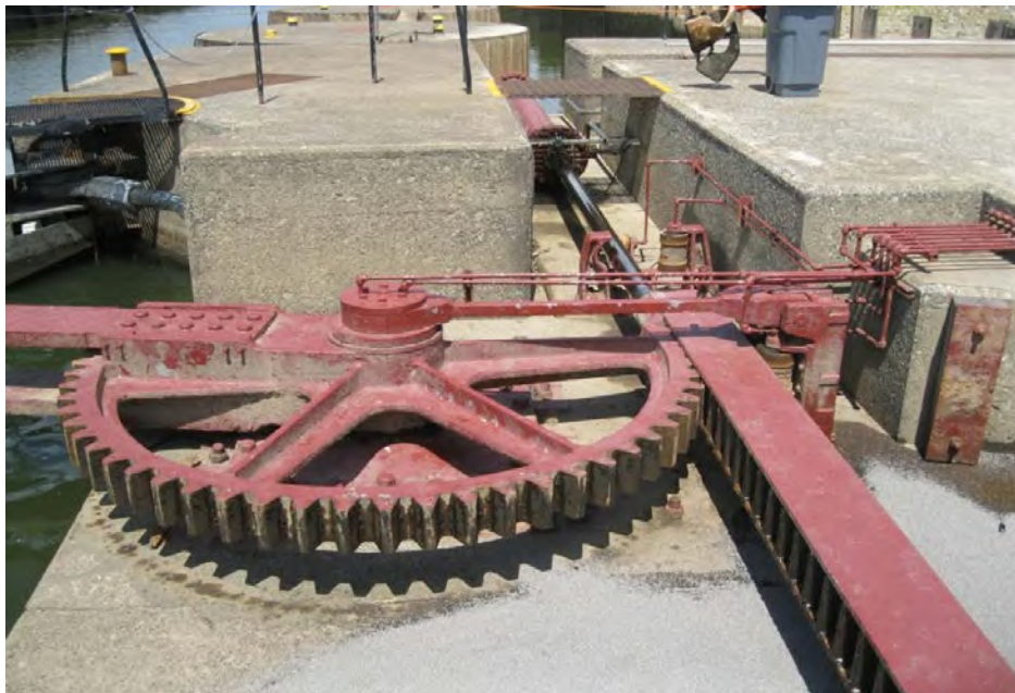
Figure 14-3. Sector Gear and Rack (Rack and Pinion).
