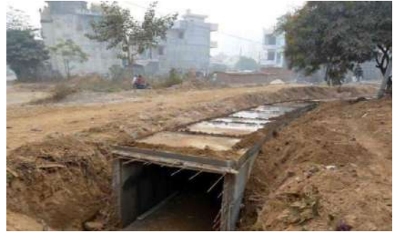
Figure 11.7: Box drain
