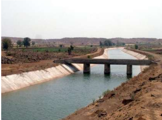
Figure 5.13: Concrete Channel
