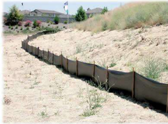
Figure 6.6: Silt Fence
