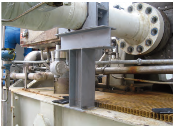
Figure 18. Check for Pipe Strain.
