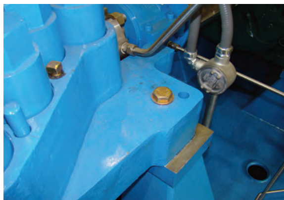
Figure 7. Overhang of Base Pad.
