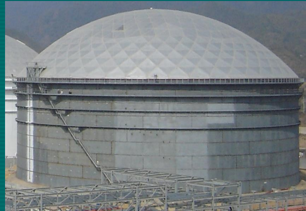
Dome Roof Tank
