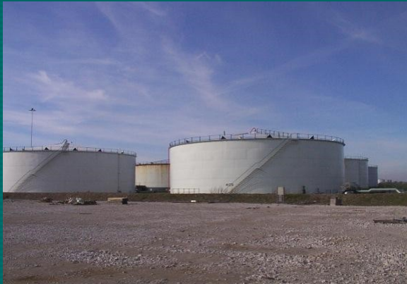
Cone Roof Tank
