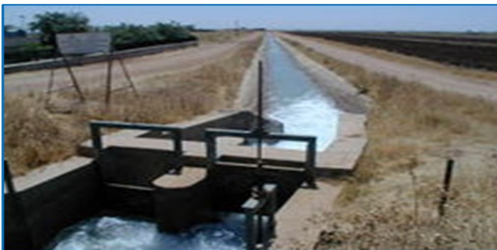
Figure (1-21): Partial (Intermediate) Regulator
