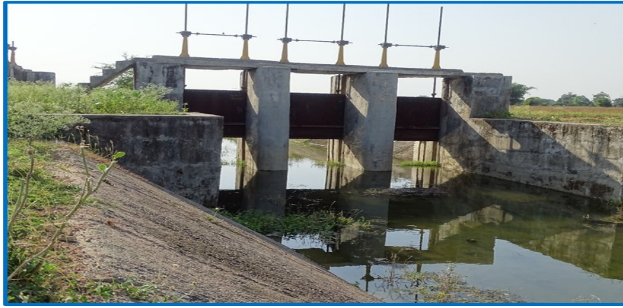
Figure (1-22): Partial (Intermediate) Regulator
