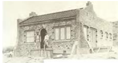
Government housing under construction in Boulder City, 1931.
