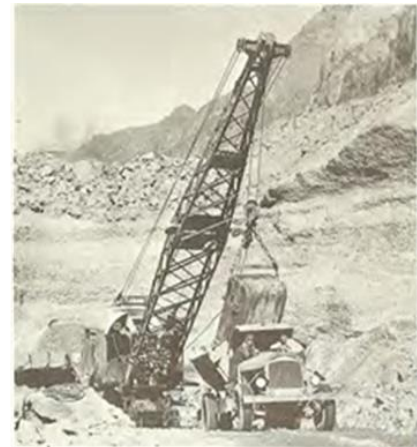
Workmen excavated thousands of tons of riverbed material to reach foundation bedrock for the dam and powerplant.
