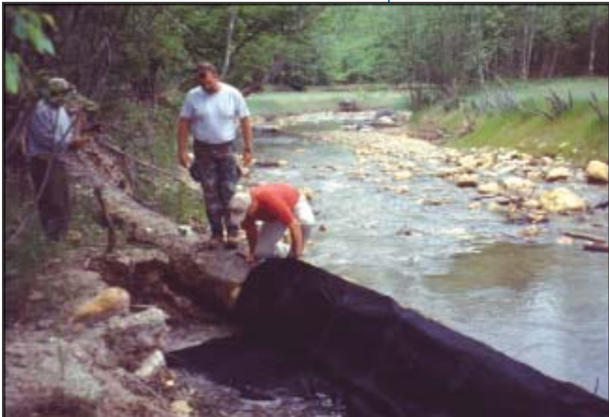
Figure 8.11 Use of geotextile fabric on the upstream side of log structure
