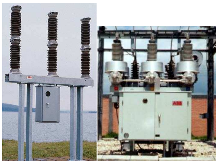
Figure 3.58: On the left a 66 kV live tank breaker and on the right a 66 kV dead tank breaker with bushing current transformers
