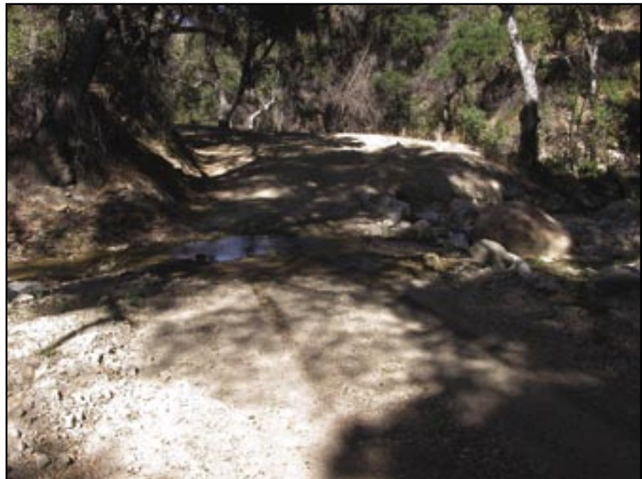
Figure 76—Low-water stream crossing replaces a 24-inch culvert.
