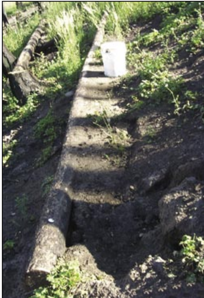
Figure 26—Contour felled LEB which has filled with sediment and then failed. Sediment trapping ability of LEBs on steep slopes is limited.
