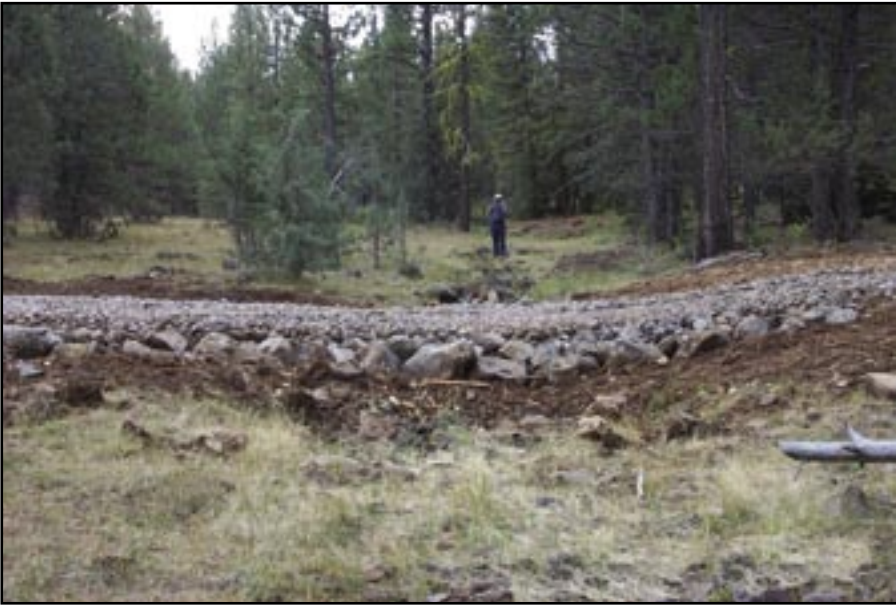
Figure 69a—Completed armored rolling dip.
