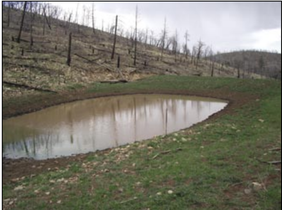
Figure 60—Small basin created to trap sediment.
