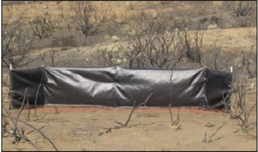
Figure 33—A recently installed silt fence.
