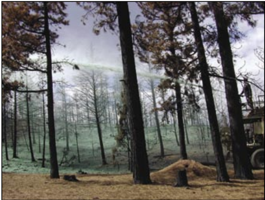
Figure 6—Ground application of hydromulch.
