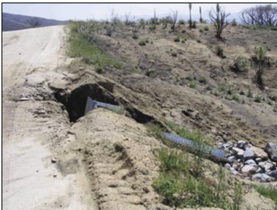
Figure 71—Failed metal roadside drain.
