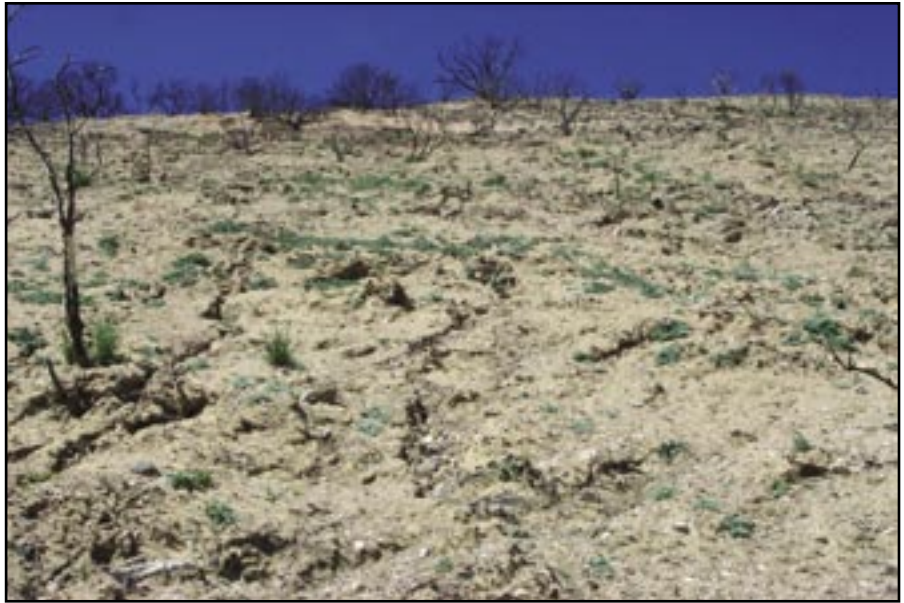
Figure 8—Treated cutslope with rilling. Longer slope lengths tend to have rilling as the runoff concentrates on the surface.
