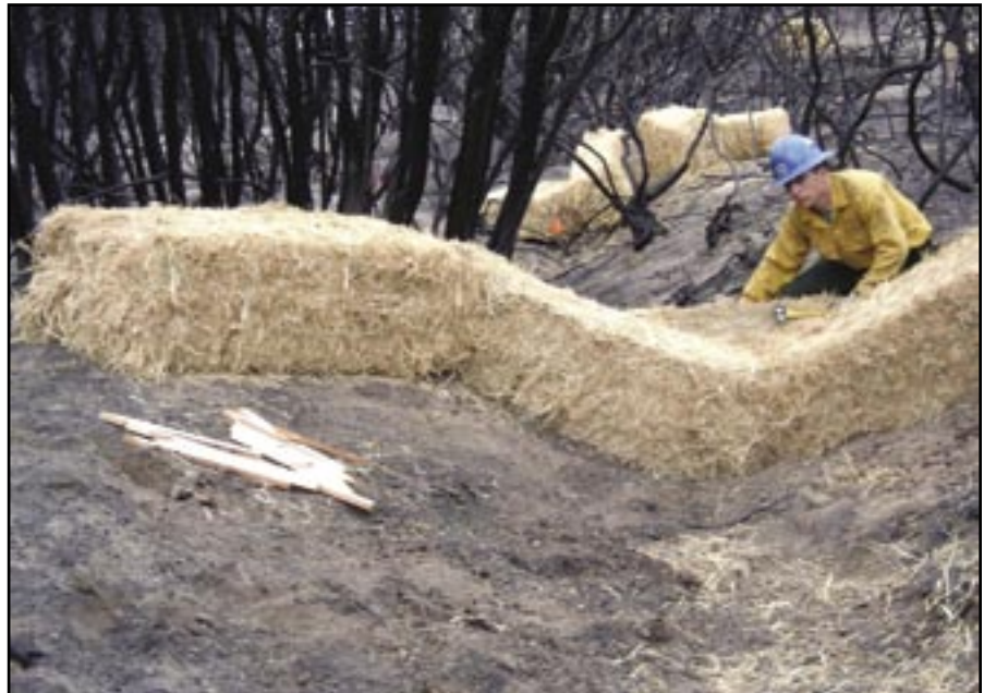
Figure 55—Install checkdams to avoid endruns.
