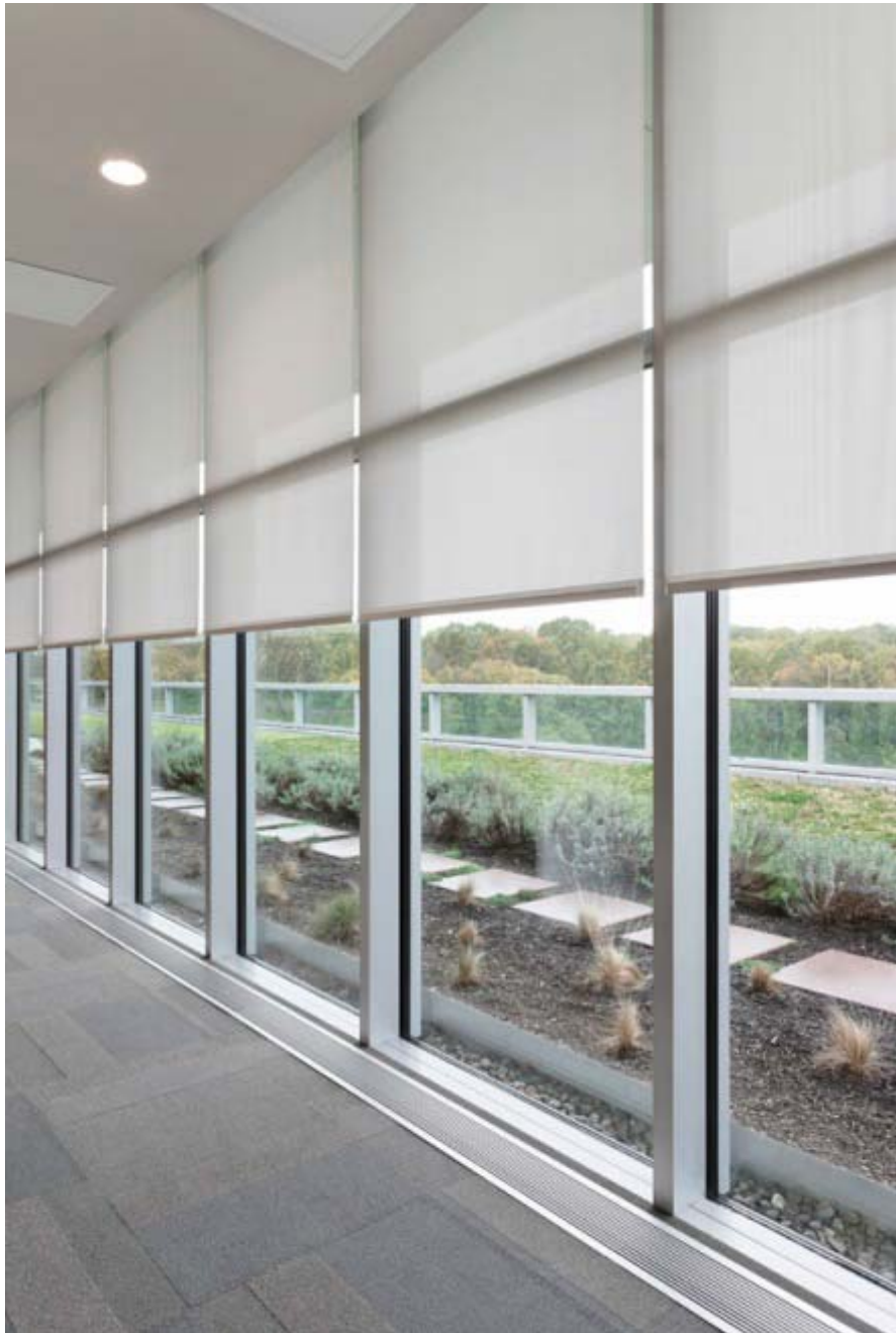
Figure 17 Example of Solar-Adaptive Shading
