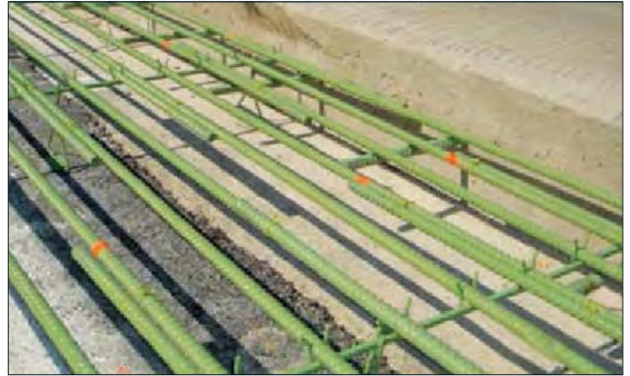
Figure 28. Longitudinal construction joint with tie bars.
