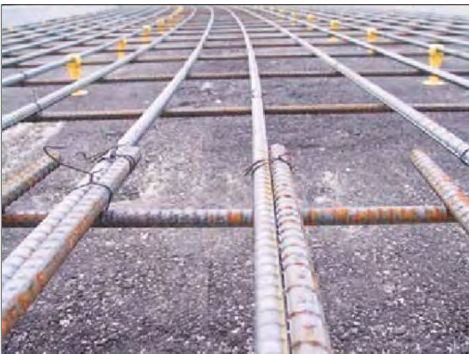
Figure 24. Lap splices.
