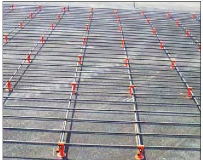
Figure 31. Steel placed on chairs (Texas).
