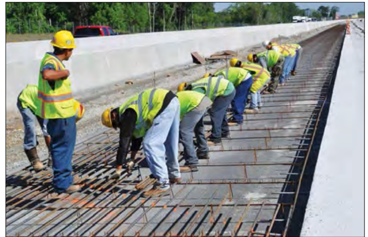
Figure 35. Placing longitudinal steel on TBAs.
