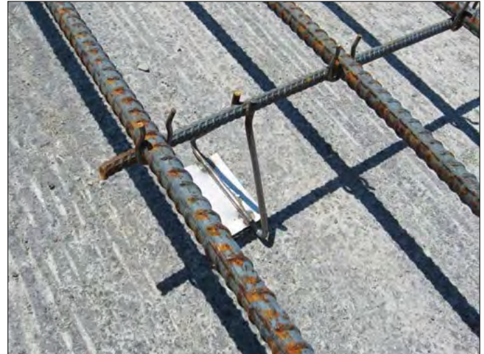
Figure 34. Transverse bar assembly (TBA).
