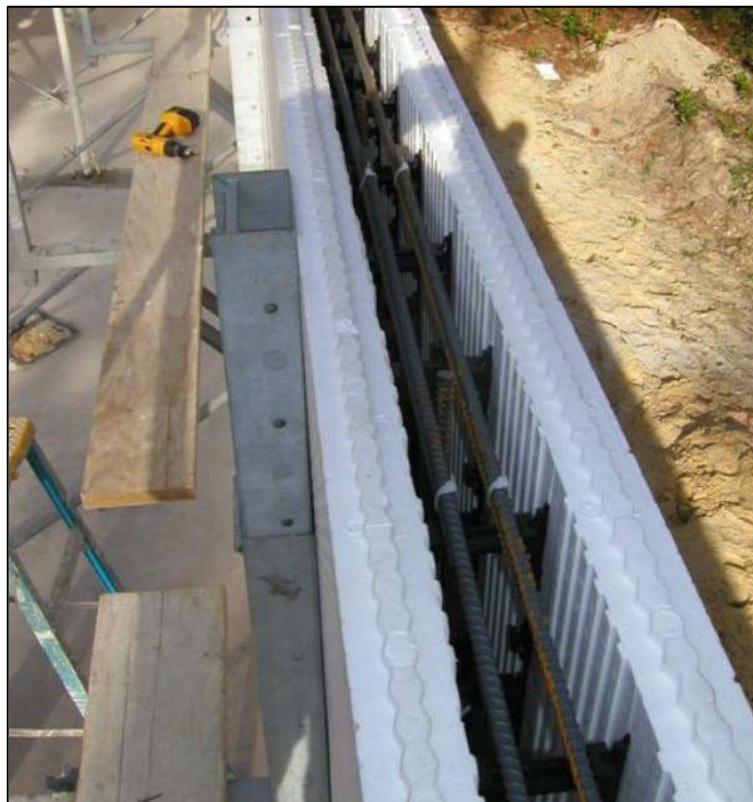
Figure 19. Insulated concrete forms before pour
