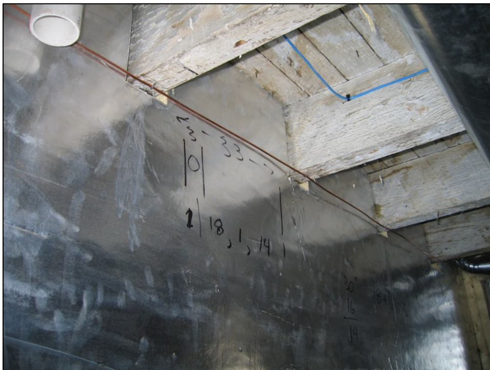
Figure 3. Foil-faced polyisocyanurate installed inside a basement wall
