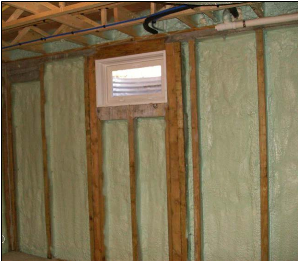
Figure 23. These pre-cast foundation panels have wood nailing strips over concrete ribs for attaching drywall. While the panels include insulation, additional spray foam has been added to these walls.
