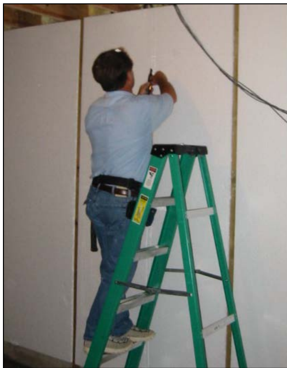
Figure 2. EPS insulation on a basement wall. Insulation will eventually be covered with drywall.
