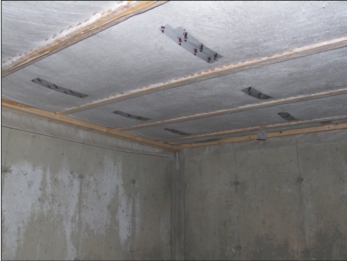
Figure 24. After air sealing, cellulose was blown into the cavities between the first-floor joists
