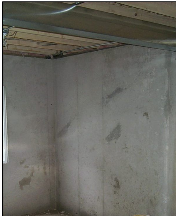
Figure 1. A basement without ceiling or wall insulation in a home built in 2001 near Chicago. Until recently, basement insulation was not required by many local codes, even in cold climates.
