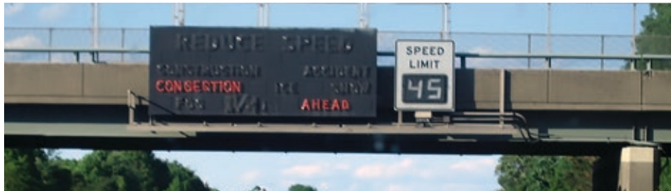
Figure 1. Photo. New Jersey Turnpike variable speed limit and variable message signing.
