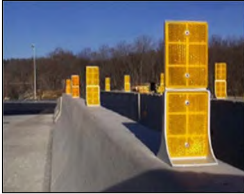
Figure 57. Photo. Delineated concrete barriers. Source: Michigan DOT.
