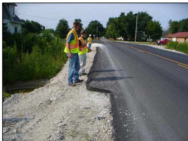
Figure 44. Photo. Shoulder paving operation.
