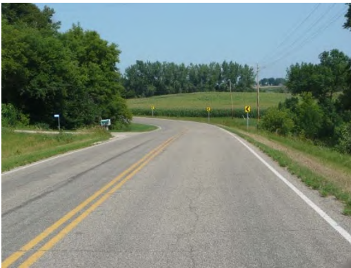
Figure 4. Photo. Delineation with chevrons. Source: MnDOT.
