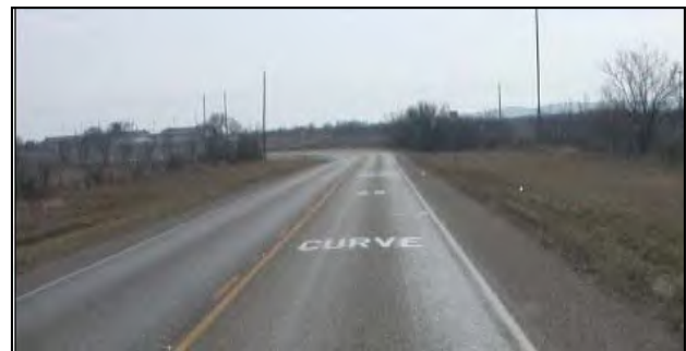
Figure 13. Photo. Pavement marking for advanced curve warning.
