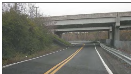
Figure 9. Photo. Edge lines.
