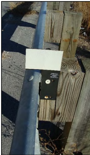
Figure 55. Photo. Delineators held in place with post bolts and installed on post.
