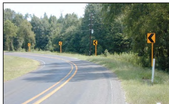
Figure 25. Photo. Chevrons assist the driver in navigating curves. Source: Texas Transportation Institute.
