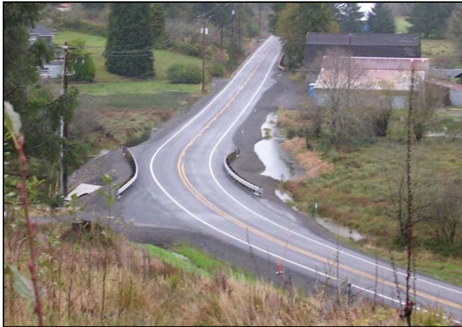
Figure 67. Photo. Intersection with paved approach.
