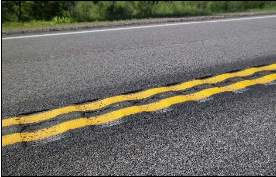
Figure 47. Photo. Milled Center Line Rumble Stripes.
