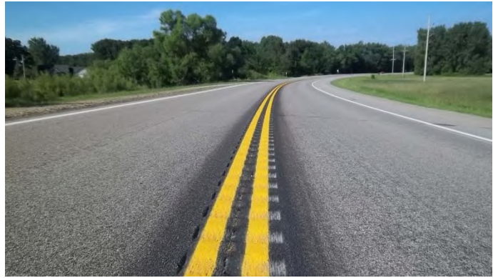
Figure 5. Photo. Centerline rumble strips.
