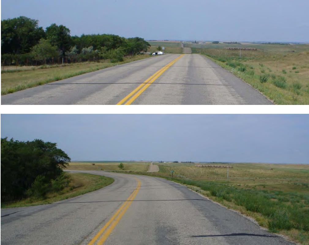
Figure 62. Photo. An example of a visual trap exists when a crest vertical curve blocks the view of the upcoming horizontal curve (top photo). What appears to be a continuation of the road in the distance is actually an intersecting roadway in the midst of a curve (bottom photo).
