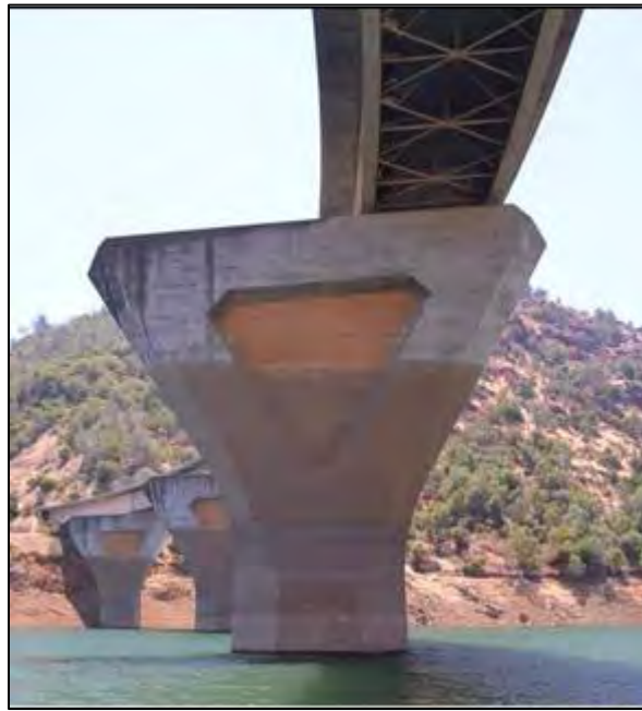
Figure 38. Photo. Northwest face of bent 4.
