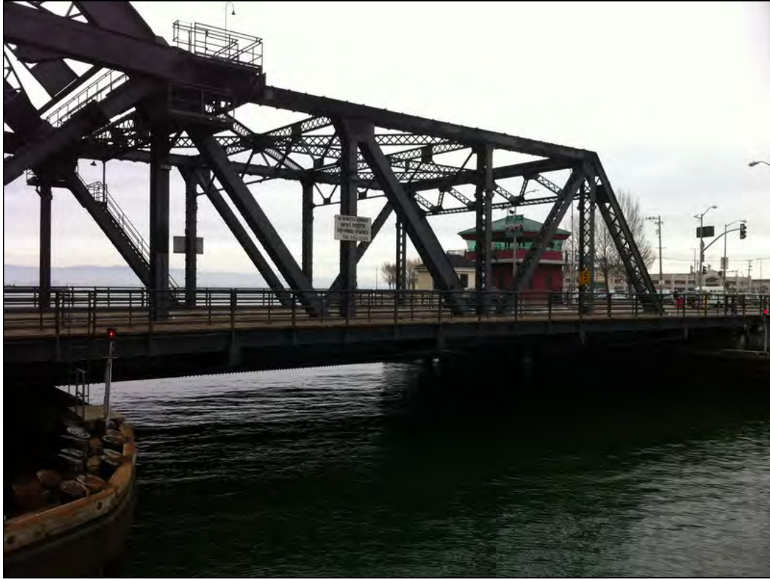
Figure 71. Photo. Third Street Bridge.
