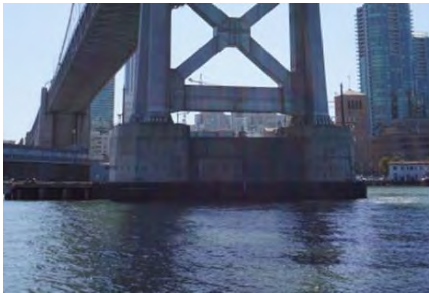
Figure 76. Photo. Pier W2 viewed from the east.
