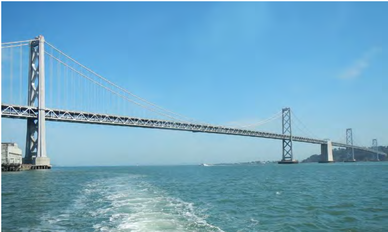
Figure 70. Photo. SF-OBB viewed from the south.
