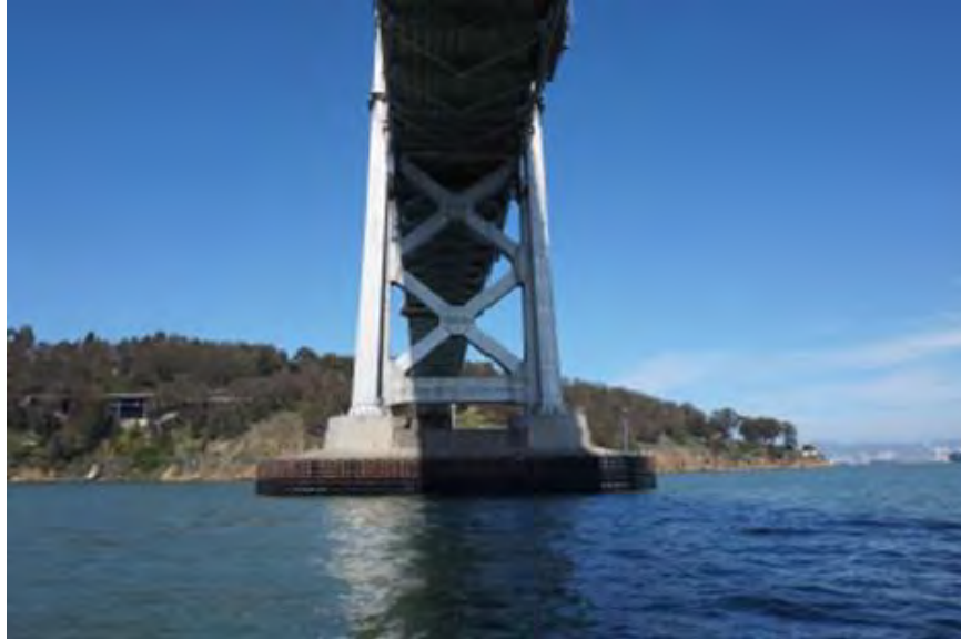
Figure 77. Photo. Pier W6 viewed from the west.
