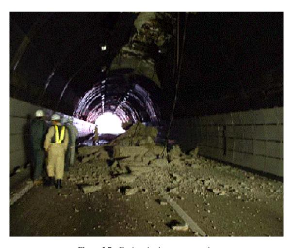
**Figure 2.7** – Earthquake damage to tunnels.
