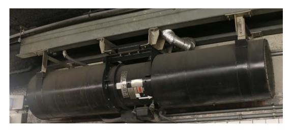
**Figure 2.2** – Emergency ventilation fan.
