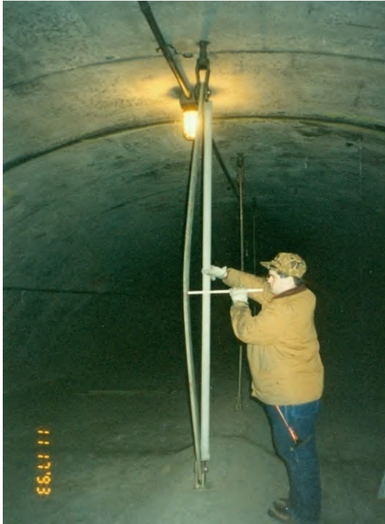
Figure 4.36 – Bent ceiling slab hanger. Note: Successive hangers are bent.
