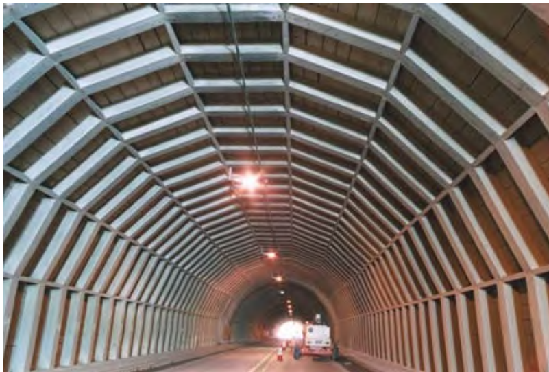
Figure 4.25 – New timber rib and lagging liner.
