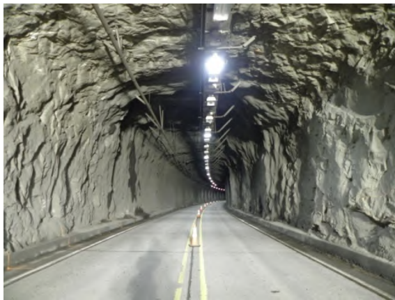
Figure 4.27 – Various unlined rock tunnels.
