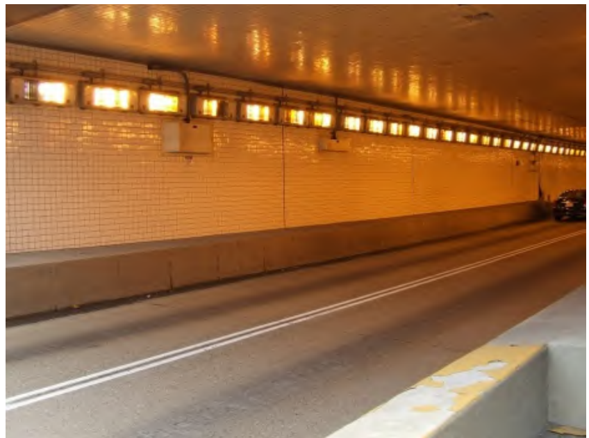
Figure 4.81 – Ceramic tile finish reflecting light.
