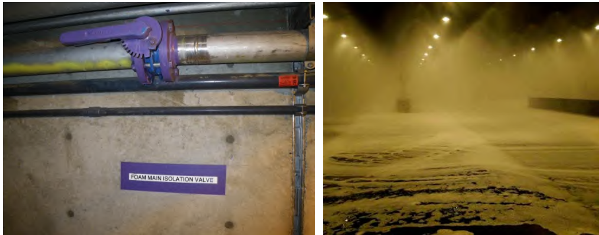
Figure 4.73 – Foam sprinkler system test.
