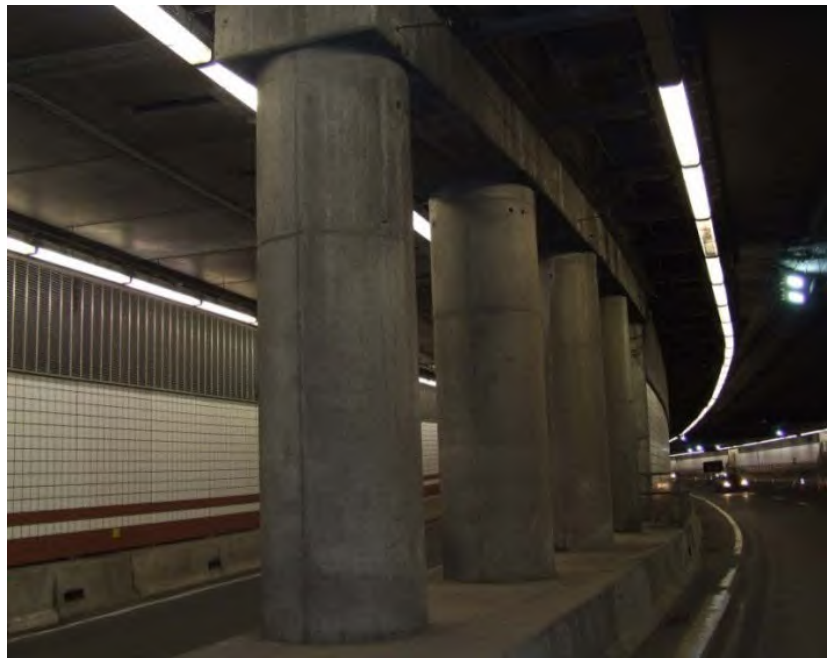
Figure 4.30 – Columns with bent cap.
