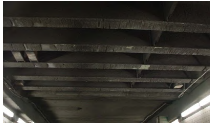
Figure 4.29 – Exposed roof girders.
