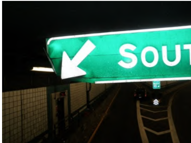
Figure 4.77 – Damaged sign.
