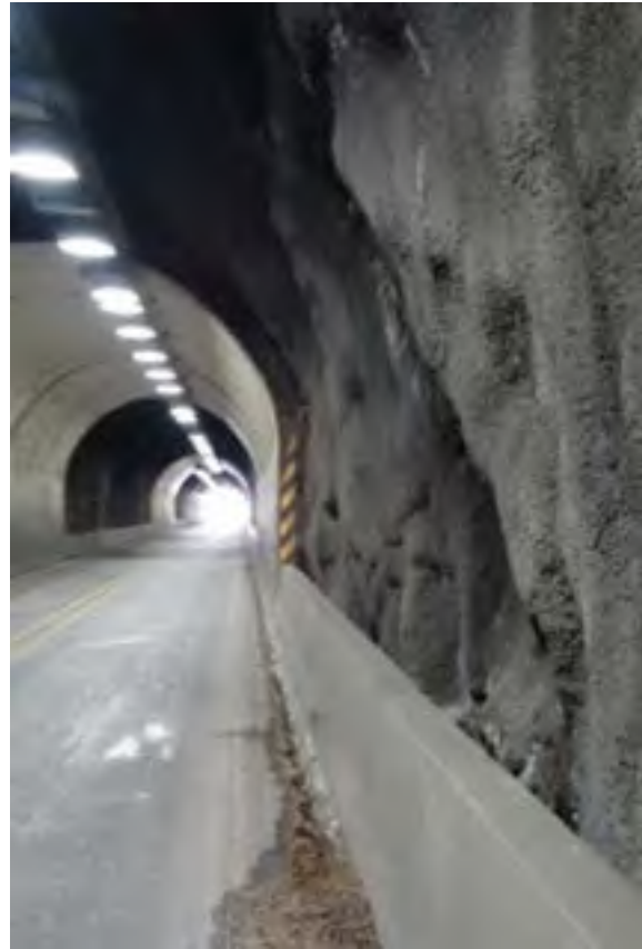
Figure 4.20 B – Shotcrete tunnel liner foreground with adjacent cast-in-place liner concrete liner background.
