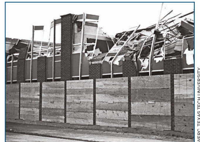
Figure 3-9 Collapsed second floor of St. Augustine Elementary School building.
