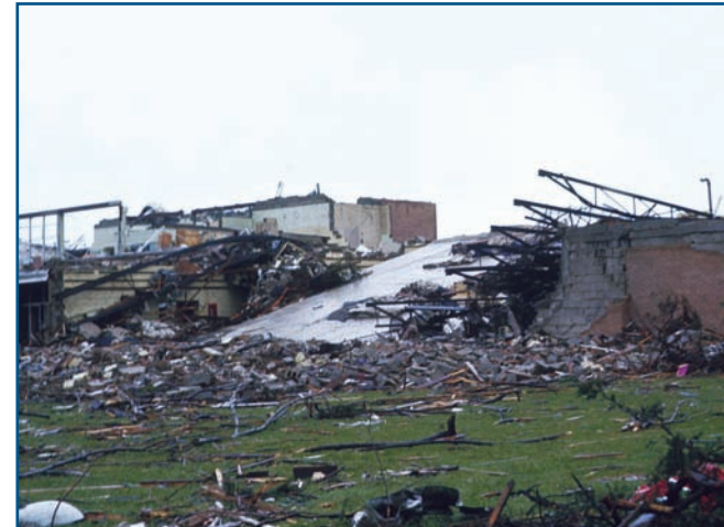
Figure 3-7 Collapsed gymnasium walls and roof, where open-web roof joists were supported on unreinforced masonry walls.
