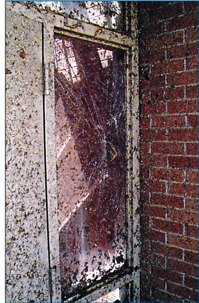
Figure 3-22 Impact performance of laminated glass. The corner of a table penetrated this laminated glass window, but the glass remained in its frame.
