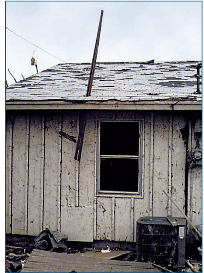
Figure 4-5 This photograph illustrates the importance of overhead protection in refuge areas. The missile shown here fell nearly straight down.
