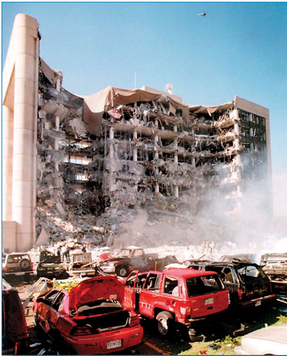
Figure 2-4 Alfred P. Murrah Federal Office Building
