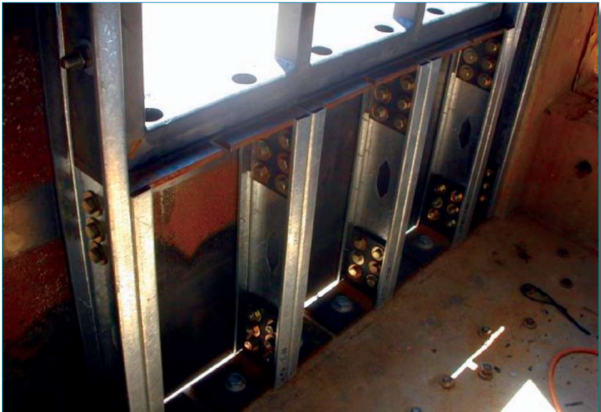
Figure 2-19 Metal stud blast wall
