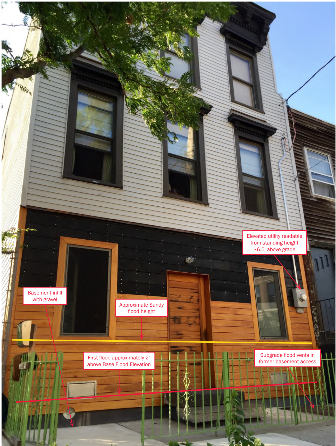
The dwelling depicted here and on the cover of this publication sustained flood damage during Hurricane Sandy in 2012. The homeowner undertook measures to make the dwelling more flood resistant in the future. The structure was retrofitted using some of the techniques featured in this publication. These techniques include elevating utilities, basement infill, and installation of flood openings. These combined measures will serve to make the dwelling much more flood resistant and have the added benefit of reducing flood insurance premiums.
