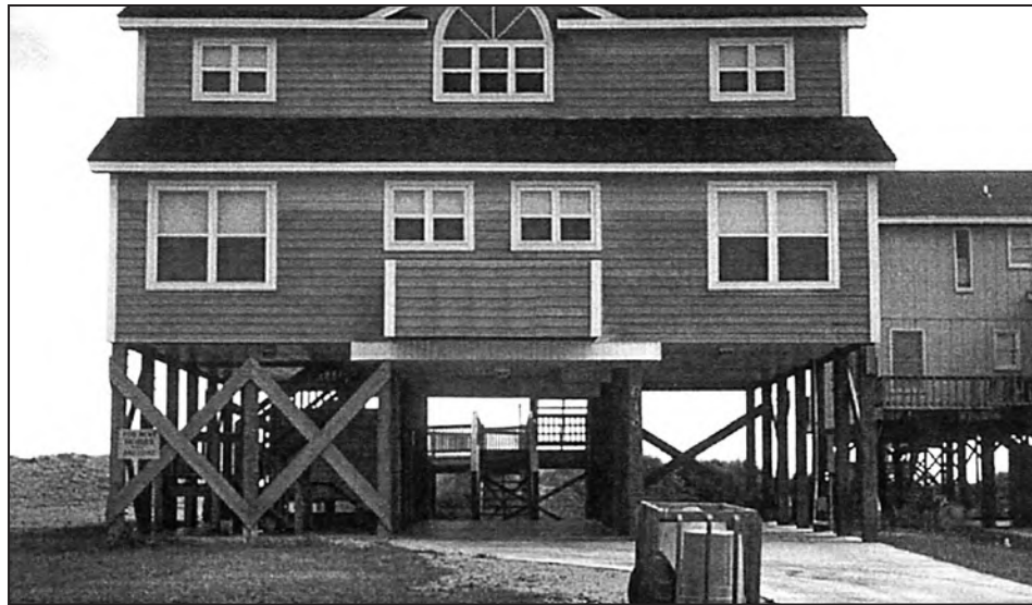
Figure 10-10. Diagonal bracing using dimensional lumber
