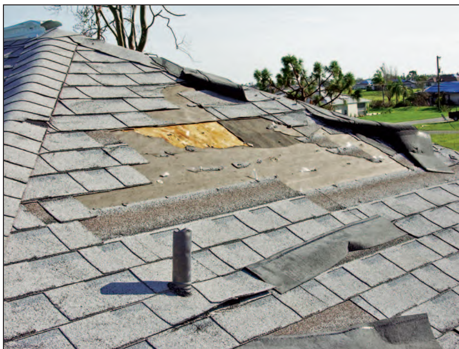
Figure 11-24. Small area of sheathing that was exposed after loss of a few shingles and some underlayment. Estimated wind speed: 140 to 160 mph. Hurricane Charley (Florida, 2004)
