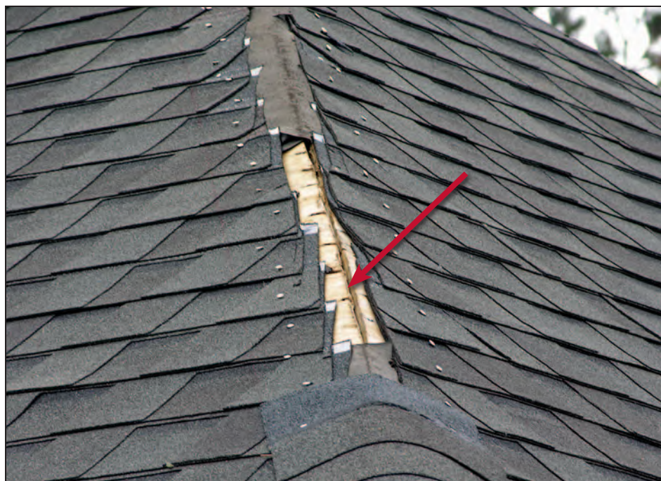
Figure 11-29. Underlayment that was not lapped over the hip; water entry possible at the sheathing joint (arrow). Estimated wind speed: 130 mph. Hurricane Katrina (Mississippi, 2005)
