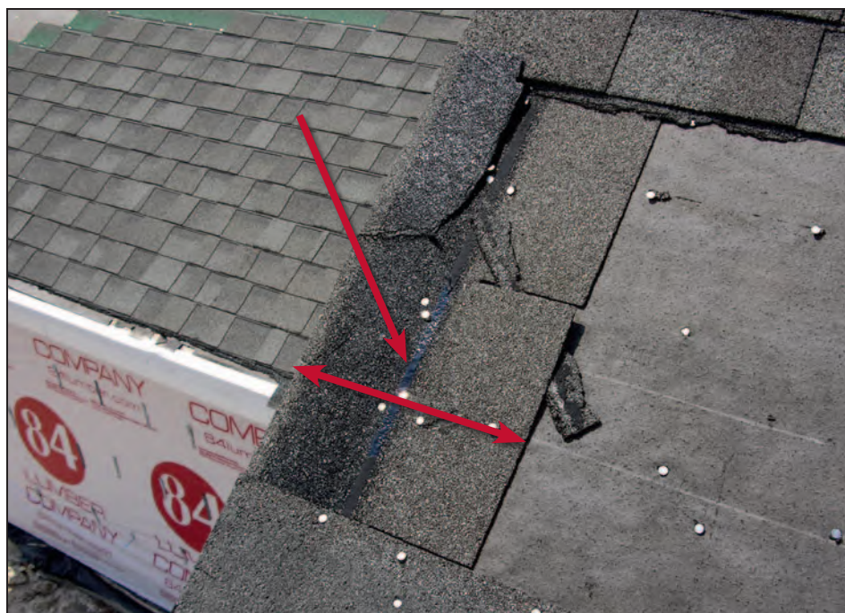
Figure 11-34. A bleeder strip (double-arrow) that was used at a rake blow-off; lack of contact between the tab of the overlying shingle and the bleeder's self-seal adhesive (upper arrow). Estimated wind speed: 125 mph. Hurricane Katrina (Mississippi, 2005)
