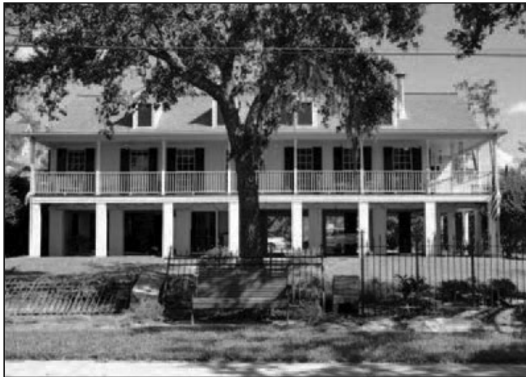
Figure 6-29. Elevation on timber piles
