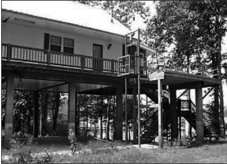
Figure 6-28. House elevated on timber piles
