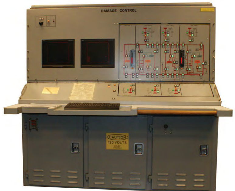
Figure 6-31 — Damage control console.
