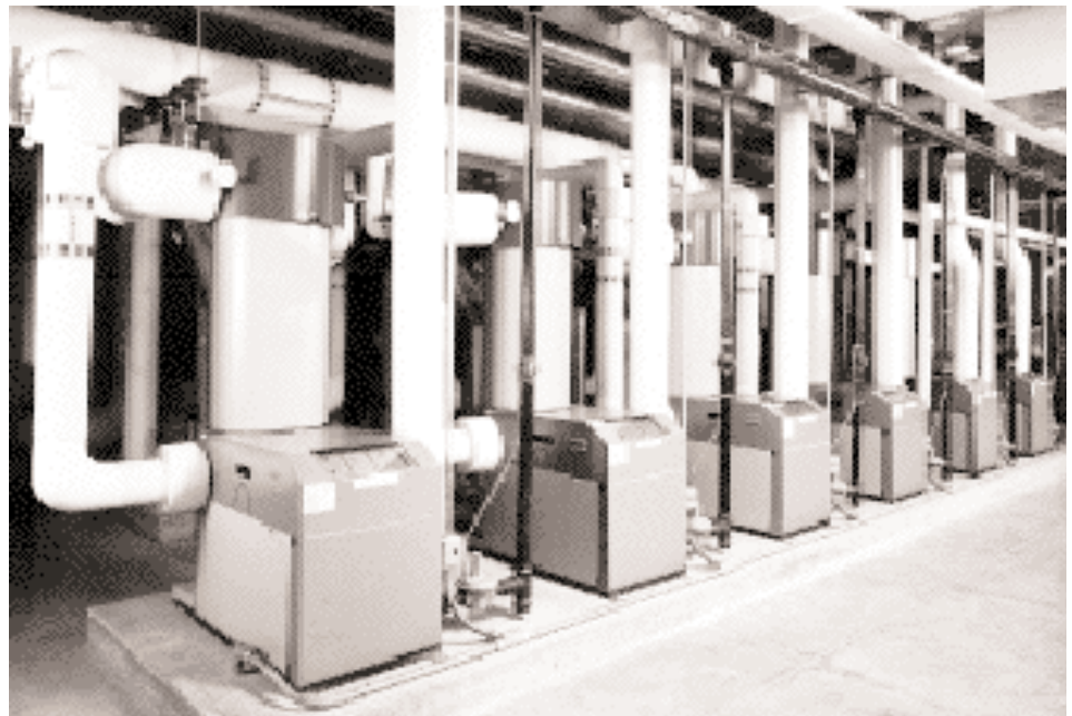
Figure 2. Typical Multi-Unit Water Heater and Hydronic Boiler Installation (photo courtesy of Aerco International, Inc.)
