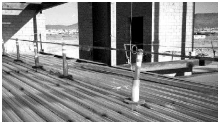
Controlled decking zone
