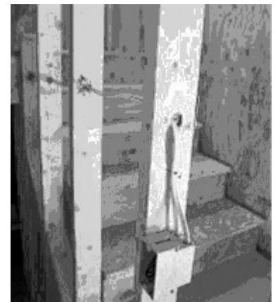
Nonmetallic sheathing helps protect wires from damage.
