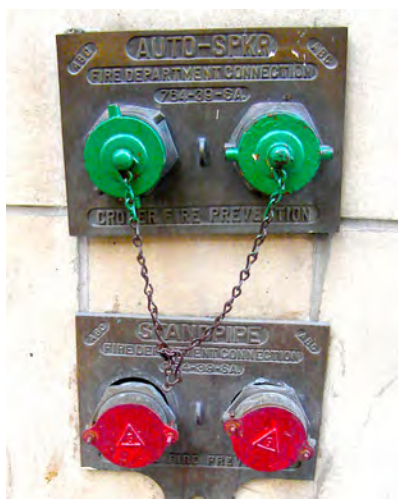
Figure 10.2. Separate sprinkler and standpipe FDCs. To feed both systems, at least one hose line must be connected to at least one inlet on each of the two FDCs.
