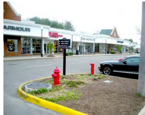
Figure 10.8. A free-standing FDC in a parking lot island near a fire hydrant.
