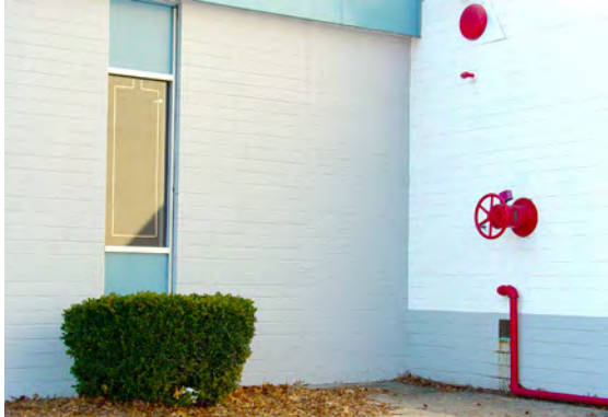
Figure 8.5. A wall control valve next to a window. Fire issuing from this window could prevent access to the valve.
