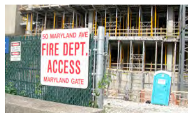
Figure 13.5. Temporary fire apparatus access.
