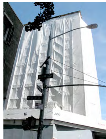
Figure 13.16. A temporary barrier covering an entire building.
