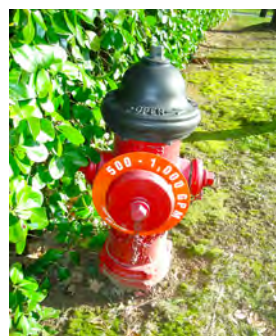
Figure 4.8. A fire hydrant with flow indicator sign.
