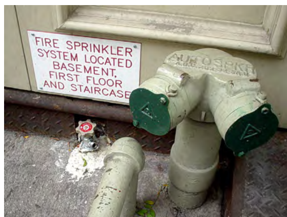
Figure 8.9. A sign indicating the areas covered by the sprinkler system that is fed by the FDC shown.
