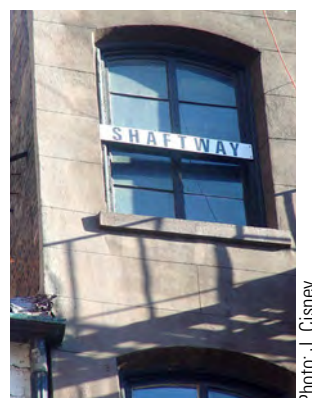
Figure 7.10. Exterior shaftway marking.
