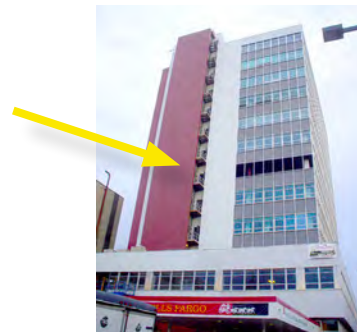
Figure 9.18. An exterior view of open air vestibules (arrow) between the stair and the interior of a building.
