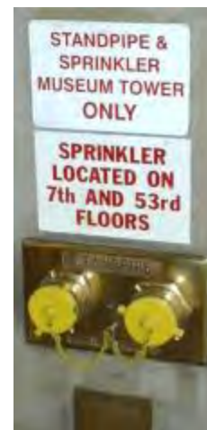
Figure 10.16. An FDC sign showing partial system coverage.
