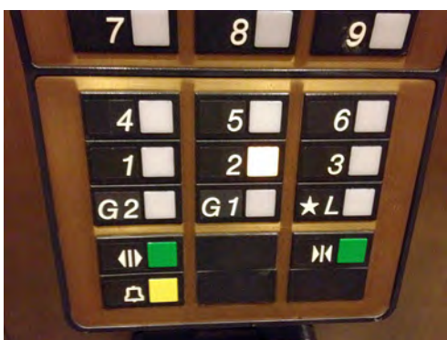
Figure 6.7. An elevator car panel in a building with both a lobby level and first floor above it.
