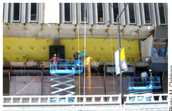
Figure 13.3. Workers on an aerial lift performing welding tasks.
