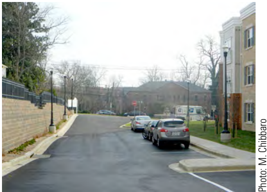
Figure 3.5. The parking spaces on the right do not reduce the width of this fire lane.
