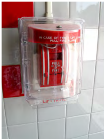
Figure 11.8. A manual pull station cover.
