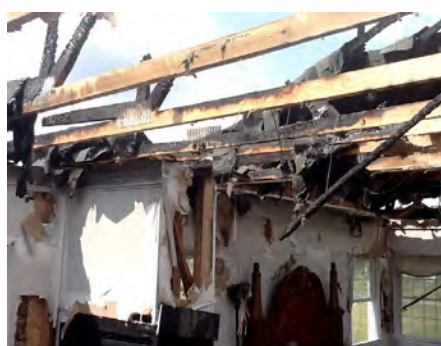
Figure 7.8. Wood trusses after an attic fire.
