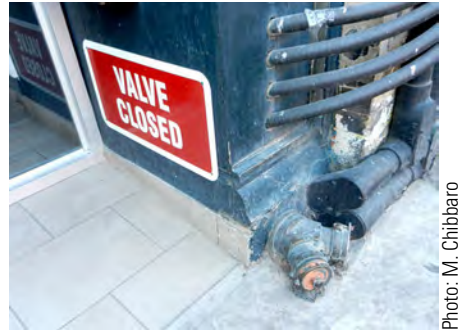
Figure 13.15. A sign next to an FDC indicating that the system valve is shut off.
