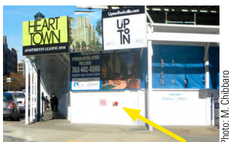
Figure 13.6. A temporary FDC (see arrow) feeding a standpipe being installed as this building rises.
