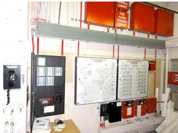
Figure 11.15. The inside of a fire command center.
