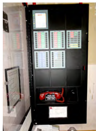
Figure 11.11. A voice alarm system panel with the door open. The microphone for live voice announcements is to the right of the red handset. The manual select switches and indicators for the different evacuation zones are shown. The red telephone handset is for the fire department communication system (see the following section) that is integrated with this panel.
