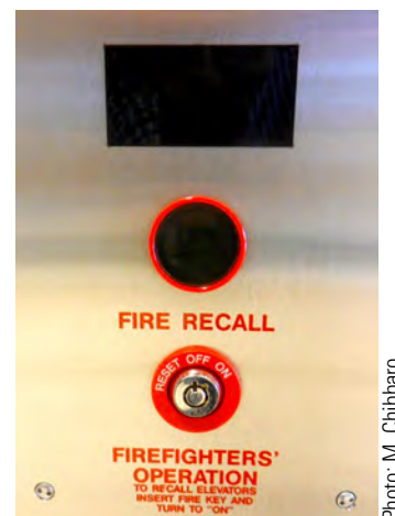
Figure 6.11. An elevator lobby switch for manual fire service recall.
