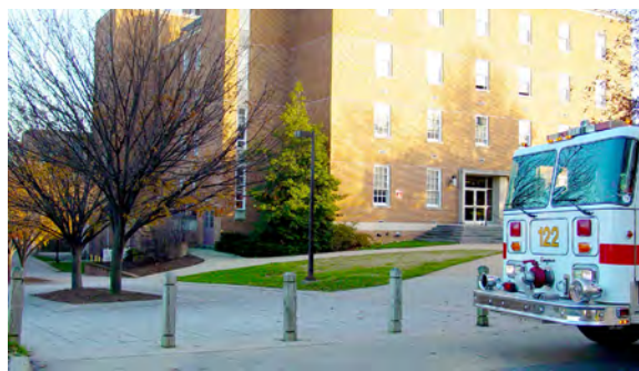
Figure 3.15. Wooden break-away bollards.
