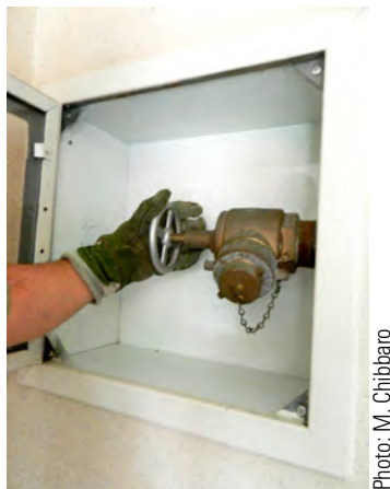
Figure 9.13. A FHC in a cabinet being checked by an inspector wearing a firefighting glove.
