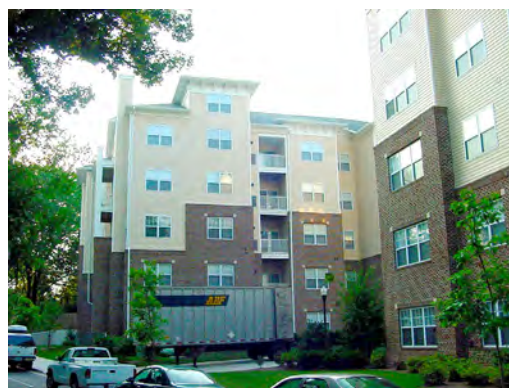
Figure 8.10. A building with six occupied levels from this vantage point. However, from a code standpoint, it is a four-story building because the top level is a loft and the bottom level is a basement mostly below grade. Its residential sprinkler system does not cover the combustible attic space or the truss spaces between floors.
