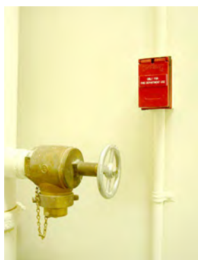
Figure 12.8. A firefighter emergency power outlet next to a standpipe fire hose connection.
