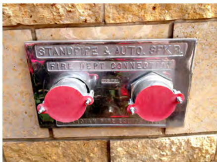
Figure 10.3. A combined sprinkler and standpipe FDC.
