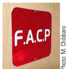
Figure 11.10 A sign on a door to a room containing fire alarm control panels (FACP).
