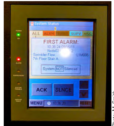
Figure 11.3 A textual-style annunciator panel with a touch-screen display.
