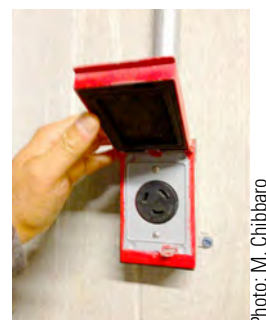
Figure 12.9. A weather-resistant outlet cover opened, showing a twist-lock type of outlet.
