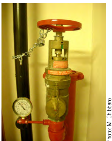
Figure 9.6. An FHC equipped with a pressure-regulating device.
