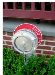
Figure 10.5. A quick-connect type of FDC.
