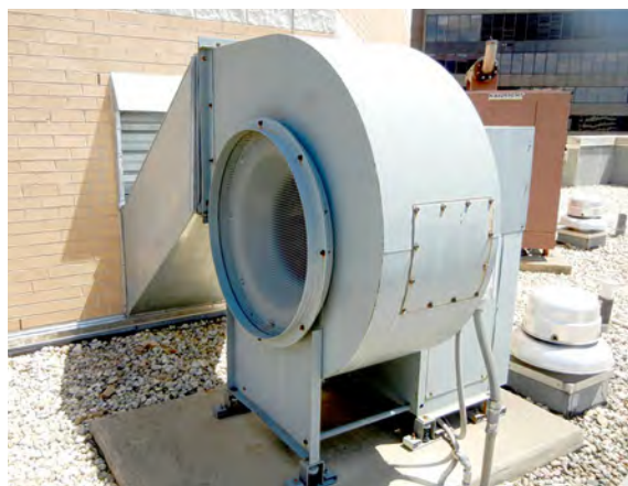
Figure 12.12. A stair pressurization fan.
