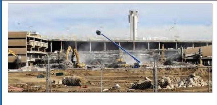
Deconstruction of Stapleton International Airport.
