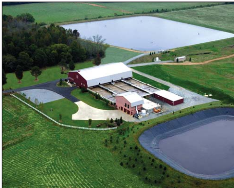
Overview of the Cauley Creek WRF Fulton County, GA
