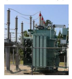
Two Winding Three Phase Transformer
