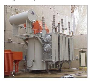
Figure 1 – Typical GSU Three-Phase Transformer.
