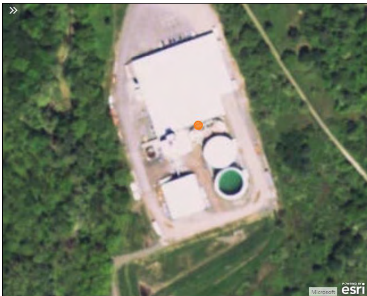
Figure 4-7. Aerial View of Eureka Standing Stone Facility
