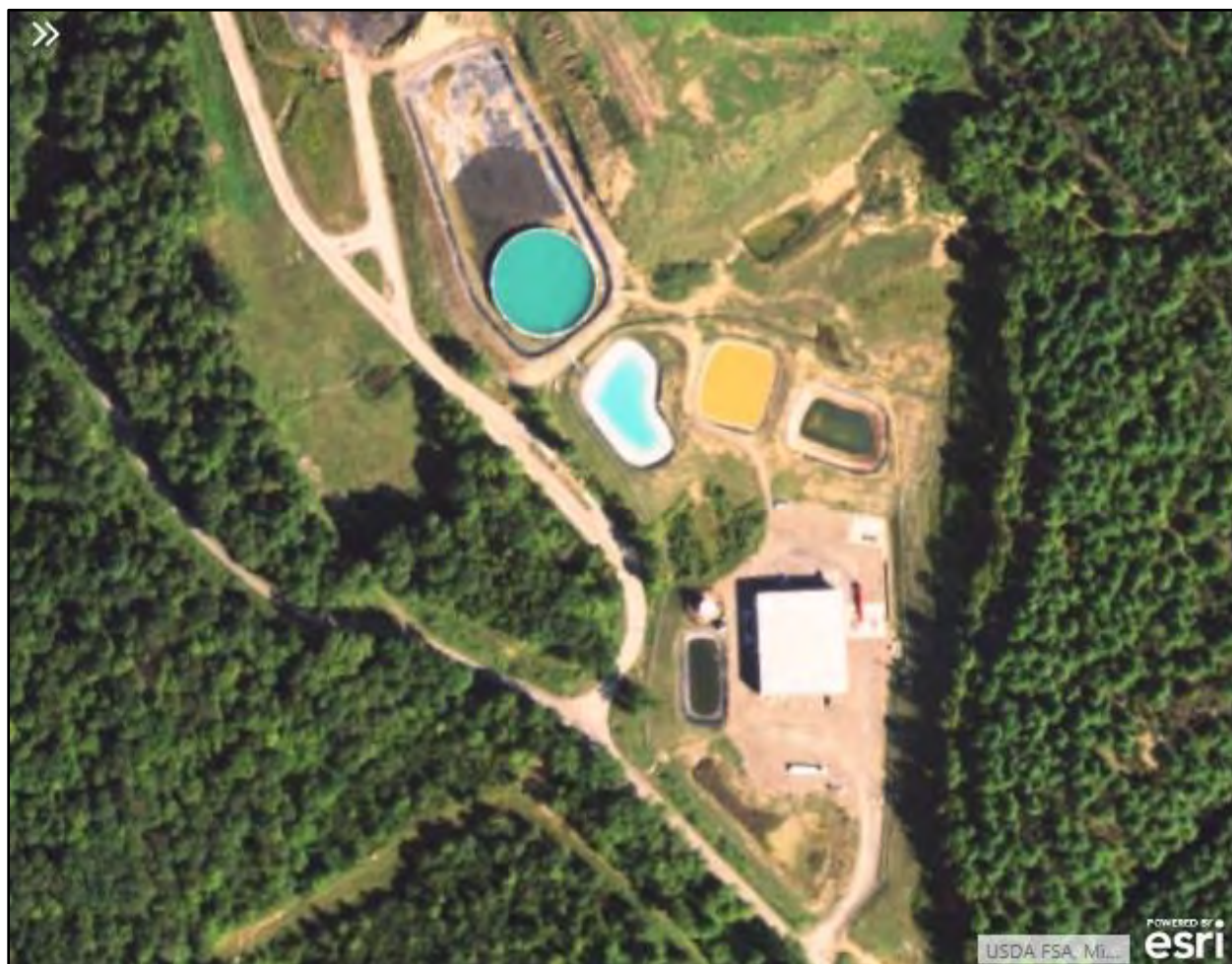
Figure 4-6. Aerial View of CAES Facility
