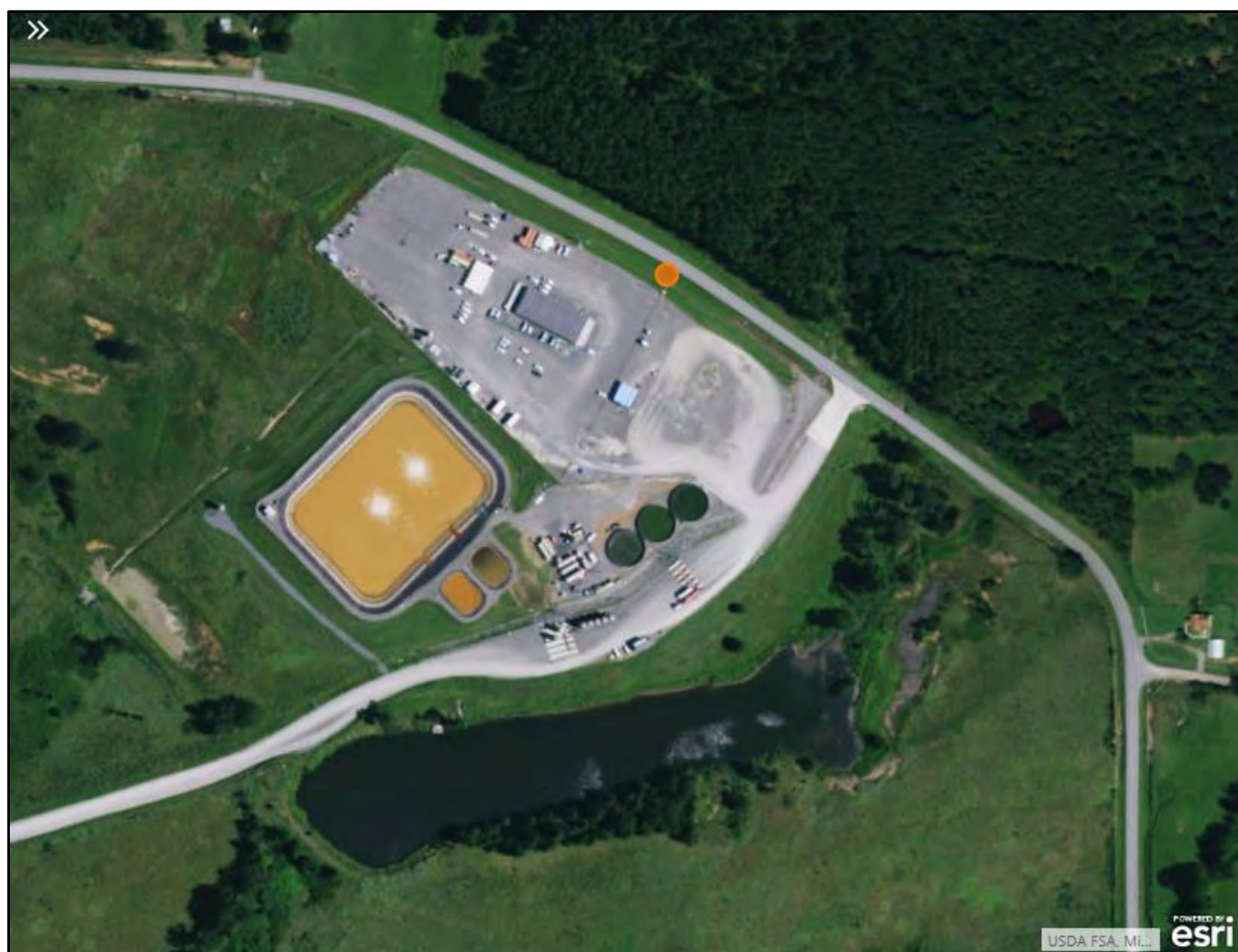
Figure 4-5. Aerial View of Judsonia Treatment Facility
