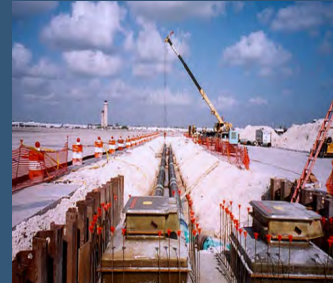
Installation of AHS piping and vaults
